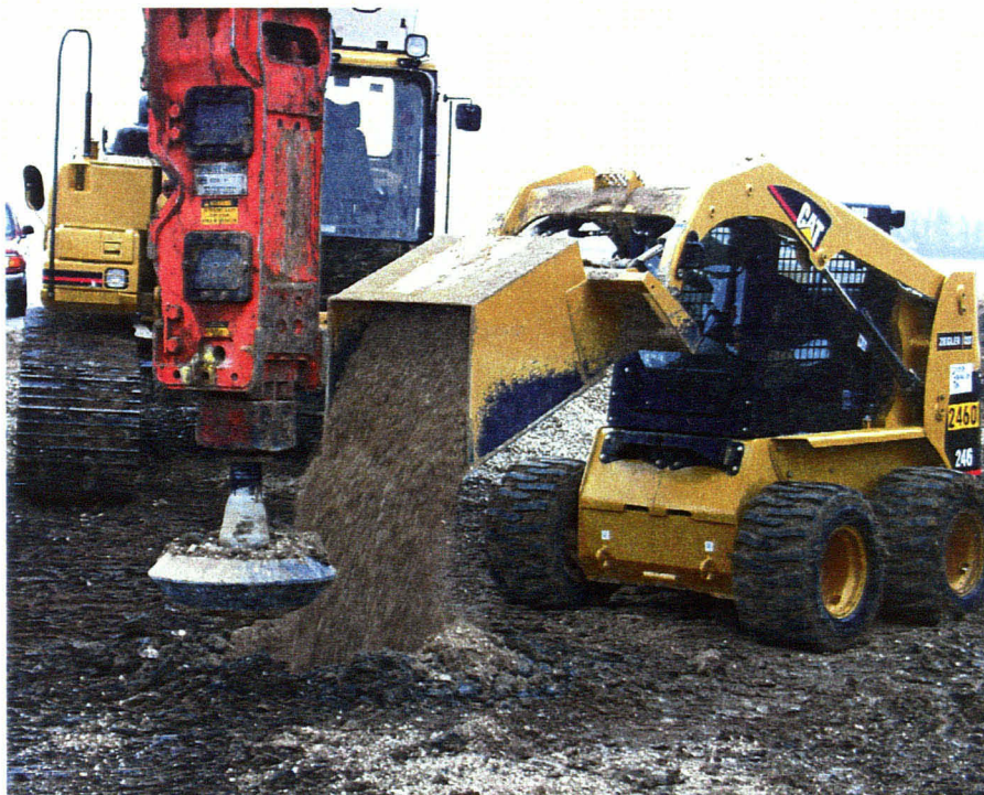
Figure 3. Aggregate placed into cylindrical cavity (beveled tamper also shown) (step 3)
