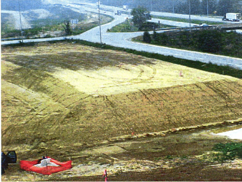
Figure 18. Ramp "C" looking from the south
