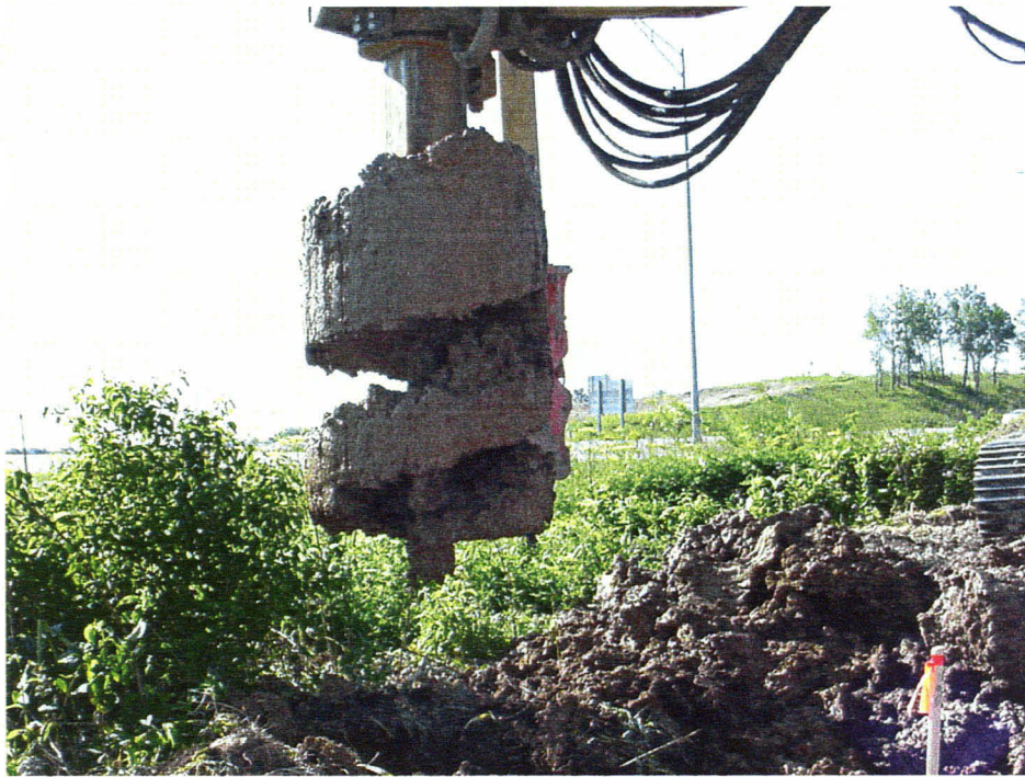
Figure 2. Auger removing saturated clay from cavity (step 1)
