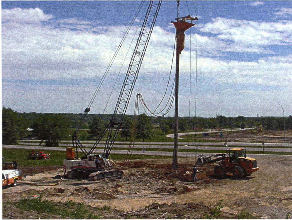
Figure 5. Vibroflot suspended from a crane (step 1)
