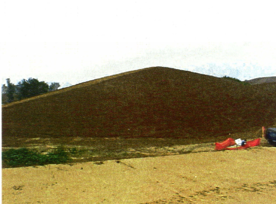
Figure 19. Ramp "B" looking from the north
